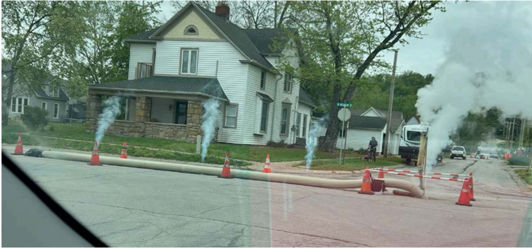
Sewer Relining Process (W Meadow St)
