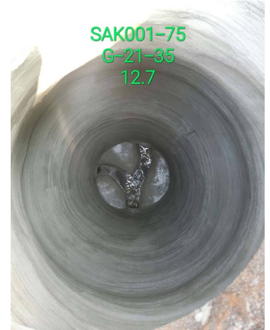
Manhole Rehabilitation (before & After)
